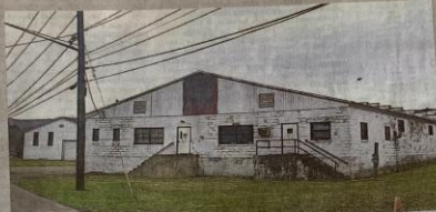
A former Agway fertilizer plant on Hammond Street in Big Flats is the target of a new citizen's group called Big Flats Defenders, which claimed the site was never remediated despite chemical contamination that has infiltrated water supplies.
